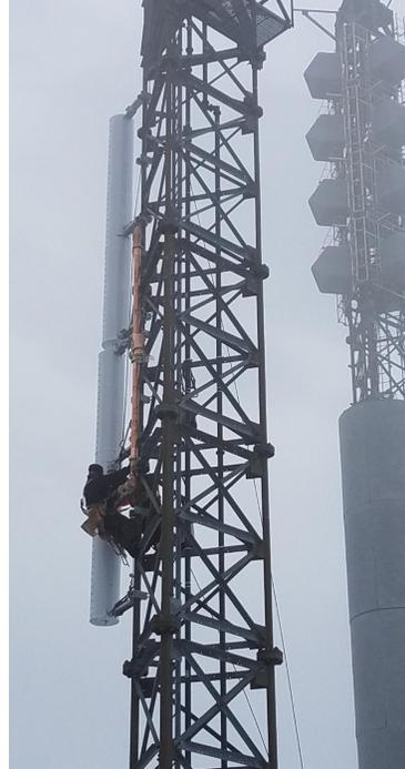
WFFF tower with the temporary antenna mounted, while the fix was being built
